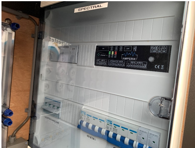
Picture 3: The Fraunhofer ITWM's energy management system goes by the name of Amperix®; myPowerGrid is a platform for microgrids and energy communities.
